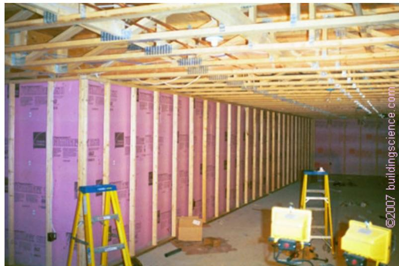
**Photograph 4:** Rigid Insulation/Frame Wall Under Construction
