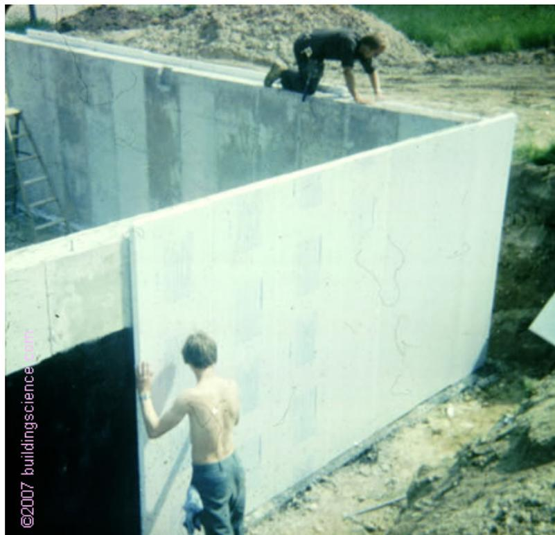
**Photograph 1:** Exterior Basement Insulation
