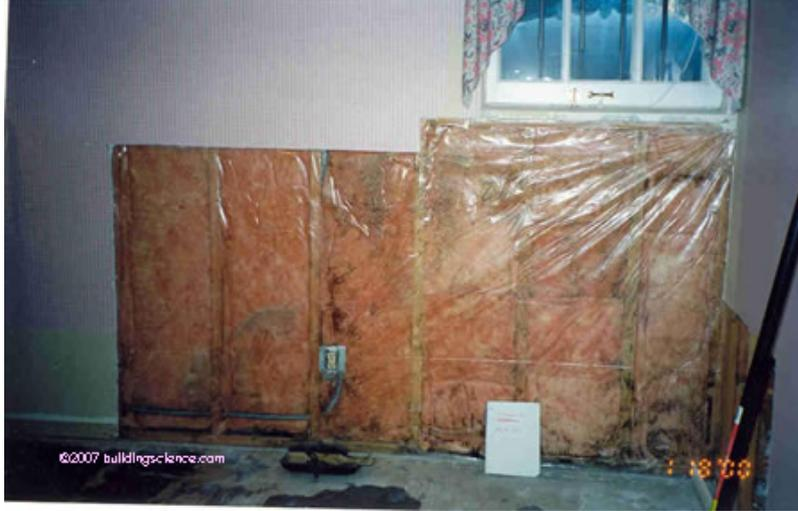
**Photograph 2:** Interior Frame Wall With Plastic Vapor Barrier
