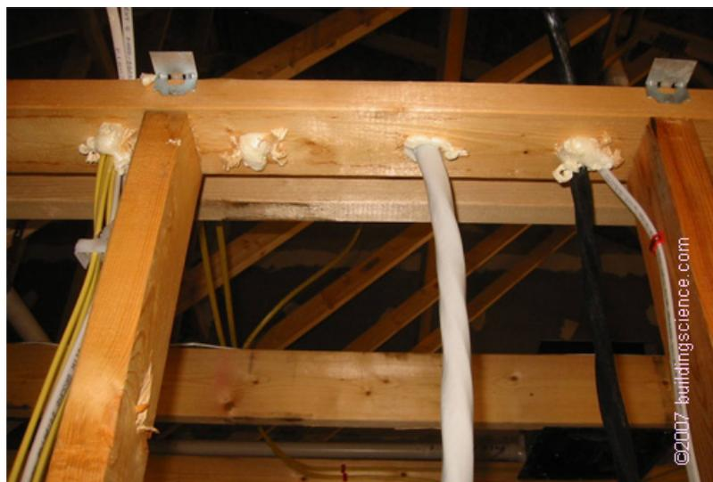
**Photograph 5:** Air-sealing with expanding polyurethane foam – much easier to do before the interior finishes are installed.
