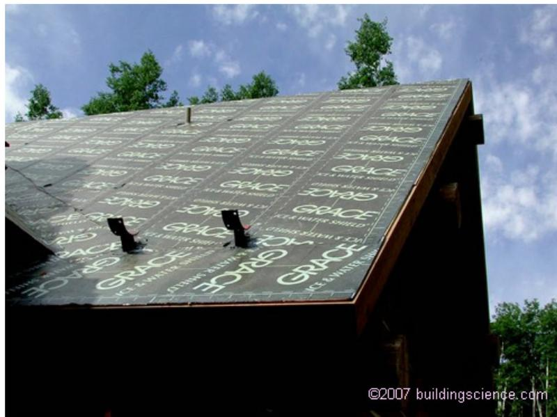
**Photograph 6:** Self-adhering membrane over the entire roof surface – an appropriate solution in some climates.
